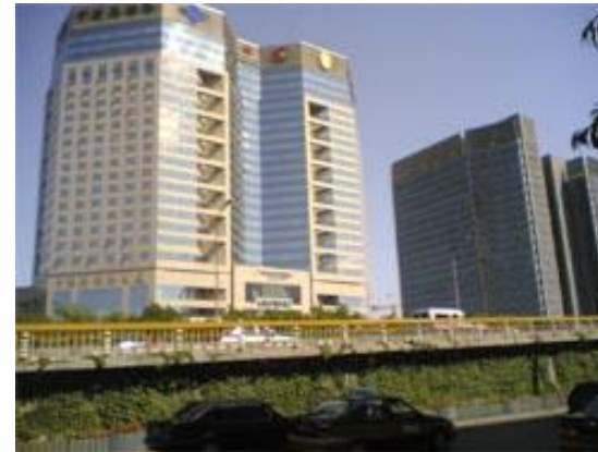
China Reinsurance Office Building, Beijing, China
